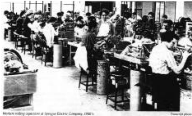
Figure 8.4: An archival photo showing electrical work at Sprague during the 1940 era.
